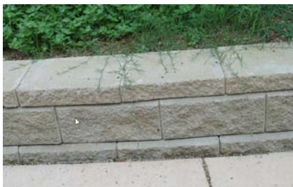
Allen Block Retaining Wall
