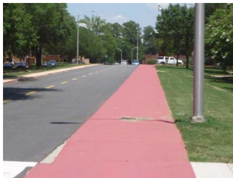
Dorms Area Concrete Bike Path
