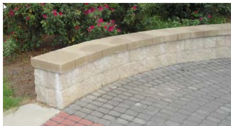
Split-face CMU retaining Wall with cap
