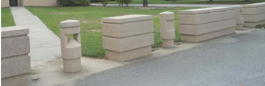
High Security Area Bollards
