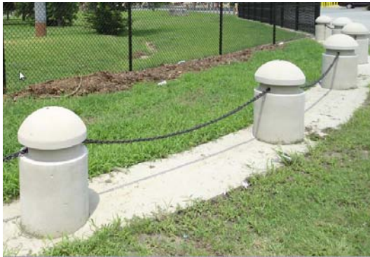
Entry Area Bollards with Steel Chain
